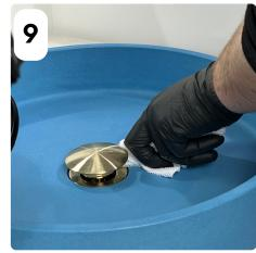
REMOVE EXCESS PUTTY, ALLOW SILICONE TO DRY FOR 24 HOURS BEFORE USE
