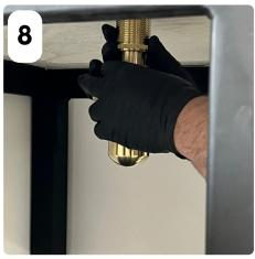
SLIDE DRAIN INTO PLACE, HAND-TIGHTEN. <u>DO NOT</u> OVER TIGHTEN
